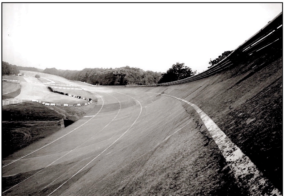
The view from the top of the Autodrom de Linas-Montlhéry (as it's officially known). The banking is nearly vertical at the top, and only vehicles doing near 100mph can hold the high line
