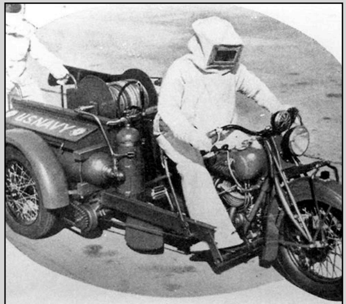
Using a custom sidecar converted this Indian motorcycle into a street sweeper and these factory built models were designed to be part of the fire department, carrying hoses, fire extinguishers, tools and firemen.
